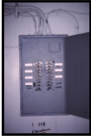
Fig. 2-9. Breaker panel.
